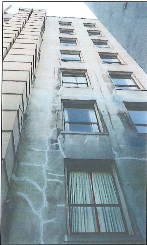
Painting walls will protect cement plaster from excessive soiling and prolong the life of sealants applied to cracks.
