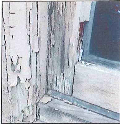
Typical conditions at penthouse wood windows include missing putty, paint loss, and splitting and separation of the sash.
