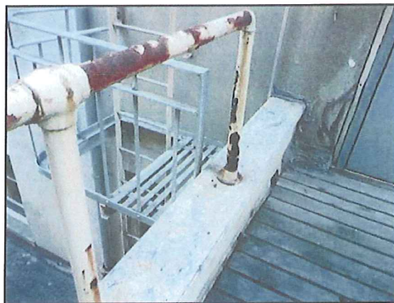
Corroding pipe rails protecting elevated walkways present a life safety hazard.
