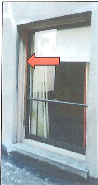
Aluminum window with unpainted wood trim
