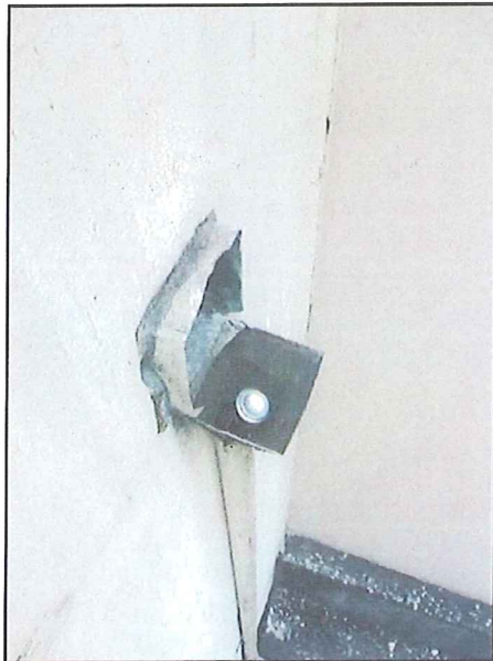
A downspout draining a 4 th floor roof is obstructed by a soft drink can.
