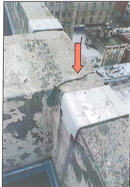
On the north parapet wall, cracks and corroding metal strap fasteners are entry points for moisture penetration that can corrode underlying reinforcing metal.
