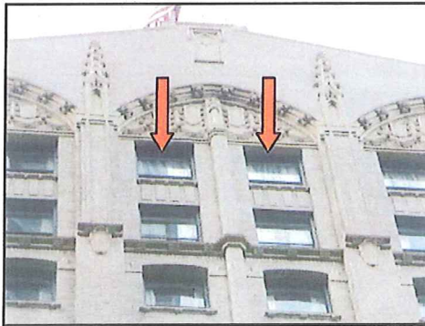
Terra cotta window headers at the 12 th floor are cracked.
