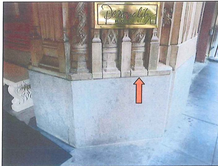
Mortar joints between the granite base and terra cotta elements are typical locations of deterioration.
