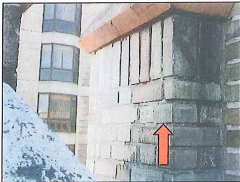
Deteriorated mortar joints are typical at front parapet wall returns.
