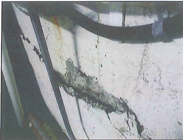
Cracked plaster is falling off a wall in the sub-basement, exposing underlying reinforcing metal to corrosion.
